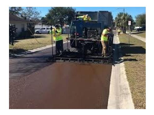
Highly Polymer-Modified (HPM) mixtures can use 7% to 8% polymer to create a more integrated polymer chain network, which improves rutting and fatigue.
