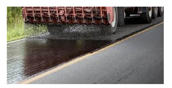
The purpose of applying a One Course Surface Treatment is to extend pavement life and arrest or retard deterioration and progressive failures.
